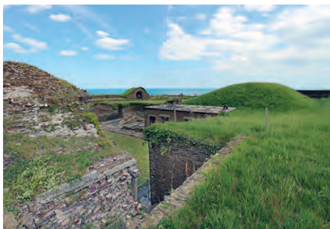
High above Dover on the Drop Redoubt ramparts. Roof of accommodation casemate to left, parade ground lower middle, small arms store on opposite rampart; the grass mound protects the magazine below. Photo Bob Clary
